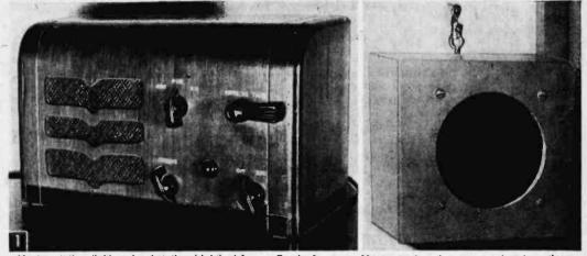
Master station (left) and substation (right) of Instant-Ready Intercom. Master station shown can select from three substation locations.
