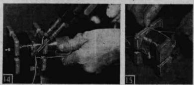
Left, at 650th turn solder a lead on end of coil wire, insulate the splice with a piece of spaghetti tubing and carry lead out slot at narrow side of form. Right, bind the coil together before removing it from the form.
