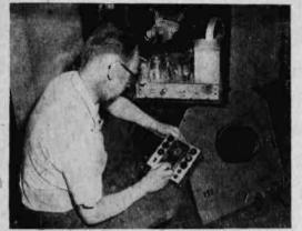
The protessional service technician usually checks tubes by substituting new tubes for those he knows from experience to require most frequent replacement. He also tests certain tubes for grid emission with the grid circuit tester. Grid emission is a very frequent cause of TV ailments and is not readily detected with general-purpose tube testers.
